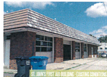
ST. JOHN'S FIRST AID BUILDING - EXISTING CONDITIONS
