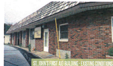
ST. JOHN'S FIRST AID BUILDING - EXISTING CONDITIONS
