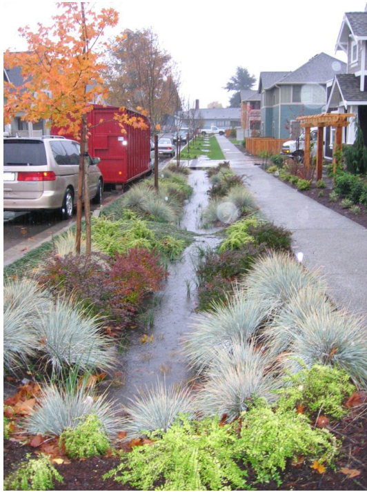
Bioswale example of stormwater best management practice
