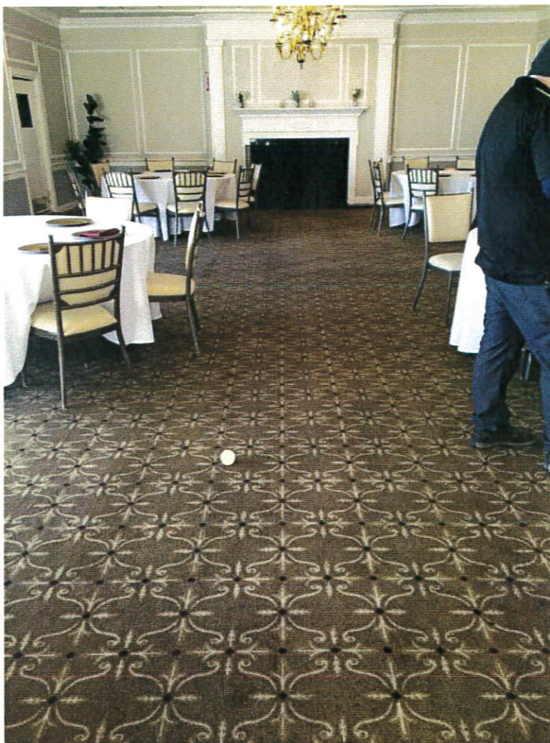
107 107-Pre-Mitigation - Dining Room Date Taken: 12/26/2022 (Zone 1) 4
