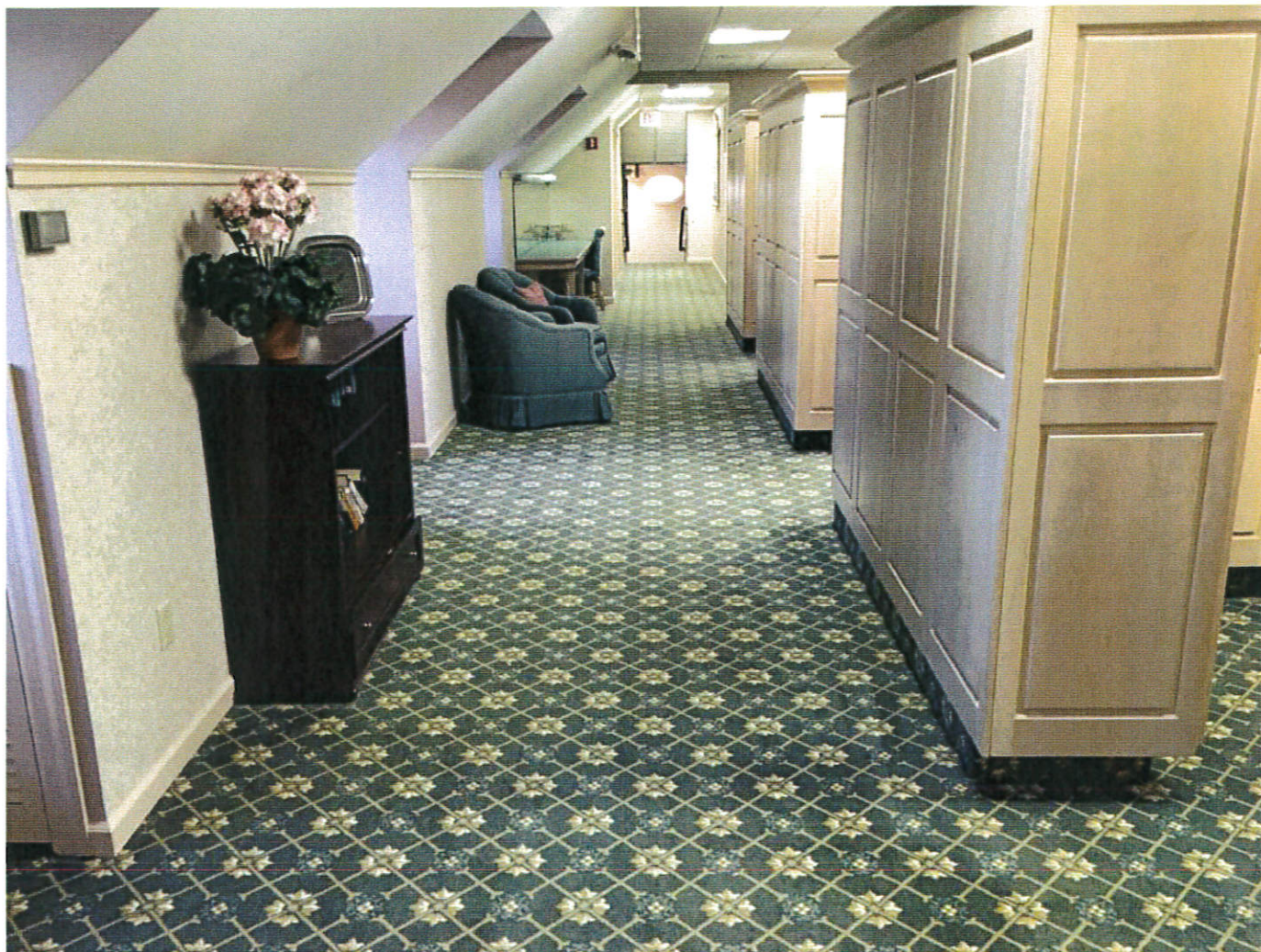
75 75-Post Mitigation - Locker room Date Taken: 12/30/2022 (Zone 1) 11
