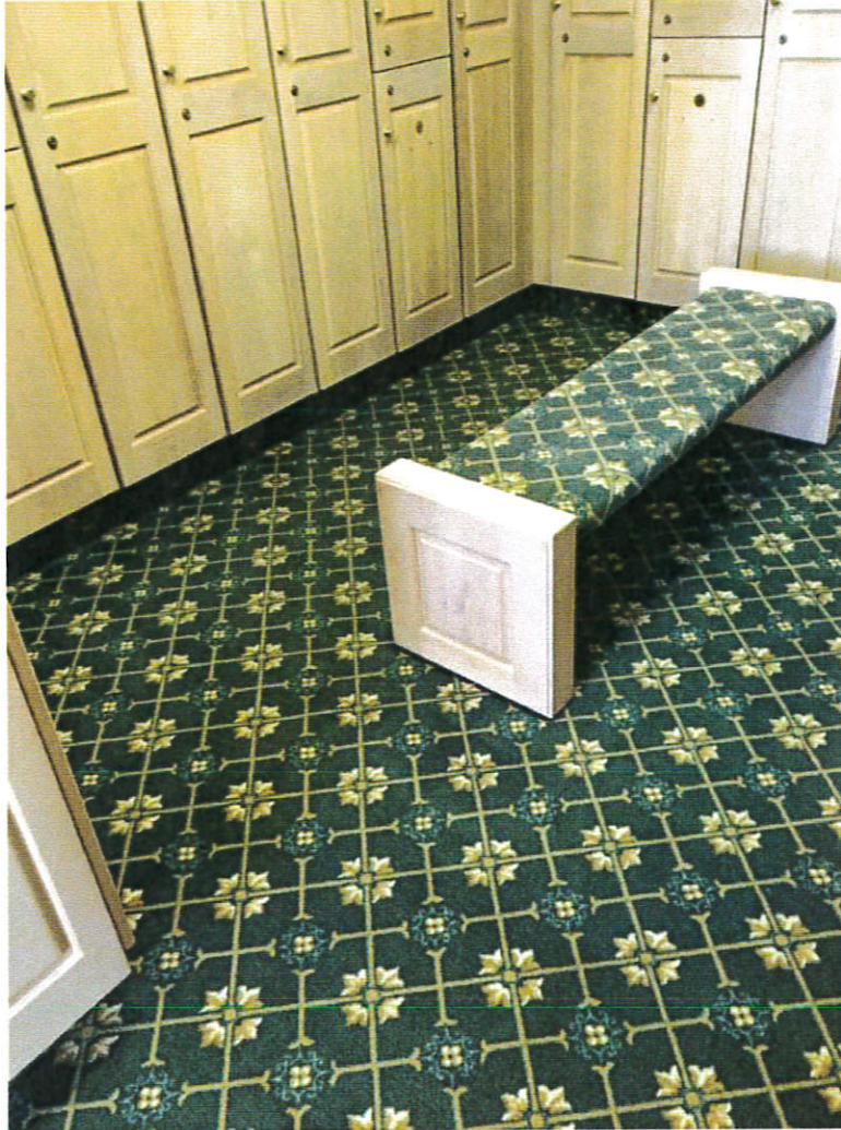
149 149-Pre-Mitigation - Locker room Date Taken: 12/26/2022 (Zone 1) 3
