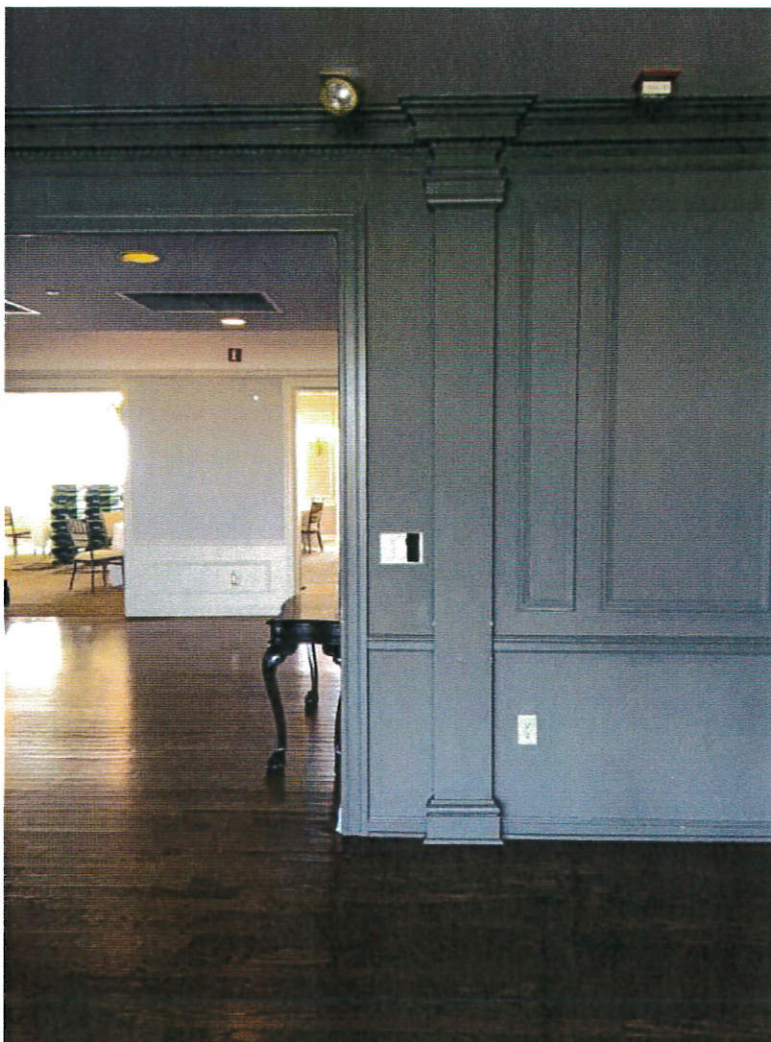
90 90-Pre-Mitigation - Ball room Date Taken: 12/26/2022 (Zone 2) 10
