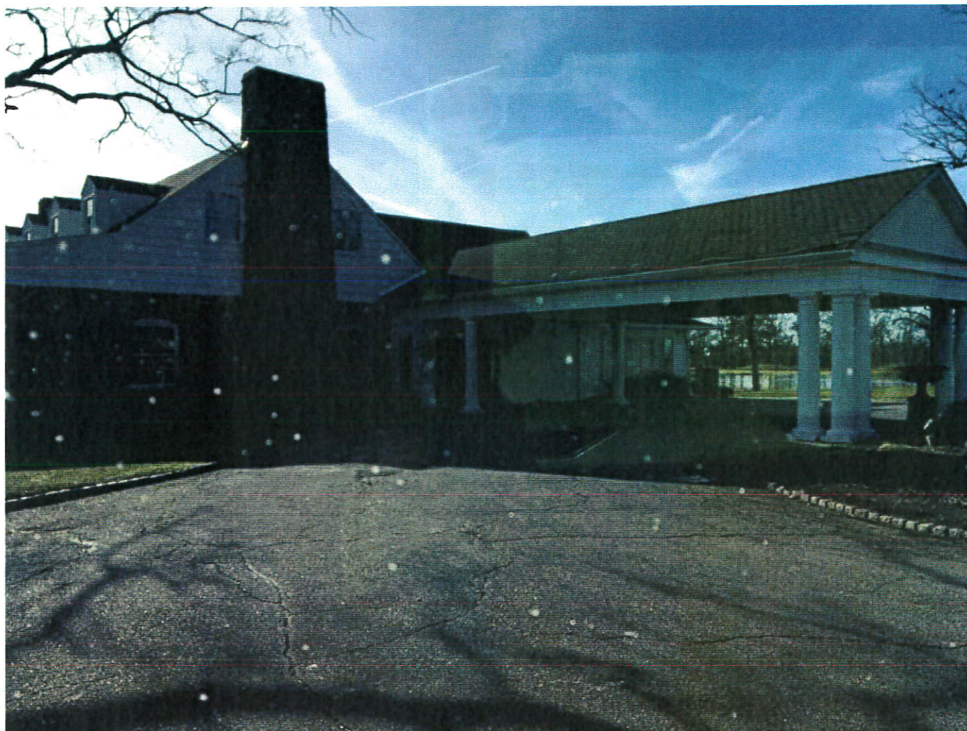
63 63-Front of Structure
