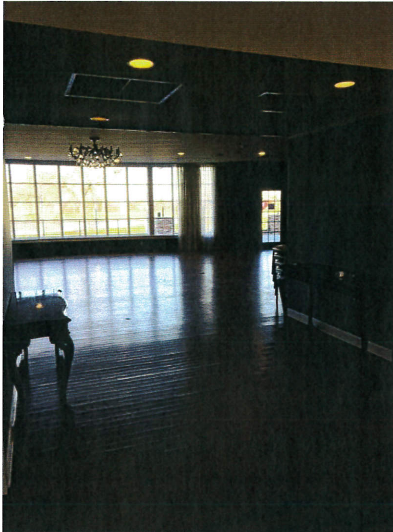
116 116-Pre-Mitigation - Foyer (Zone 2) Date Taken: 12/26/2022 12
