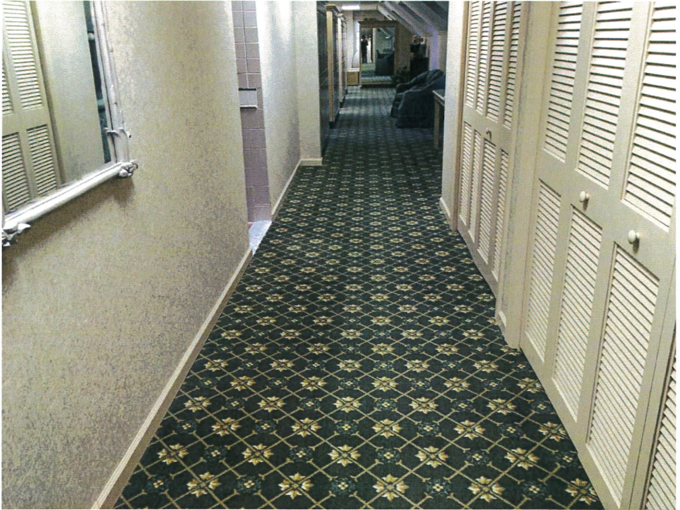
86 86-Post Mitigation - Locker room Date Taken: 12/30/2022 (Zone 1)
