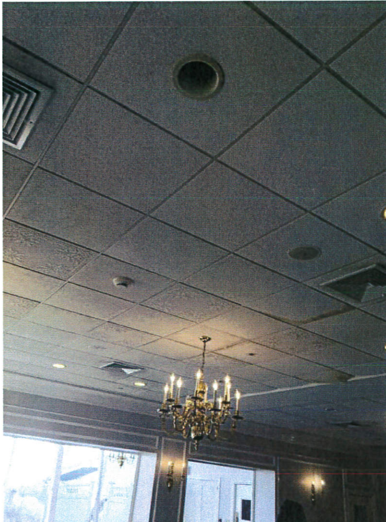
101 101-Pre-Mitigation - Dining Room Date Taken: 12/26/2022 (Zone 1) 10
