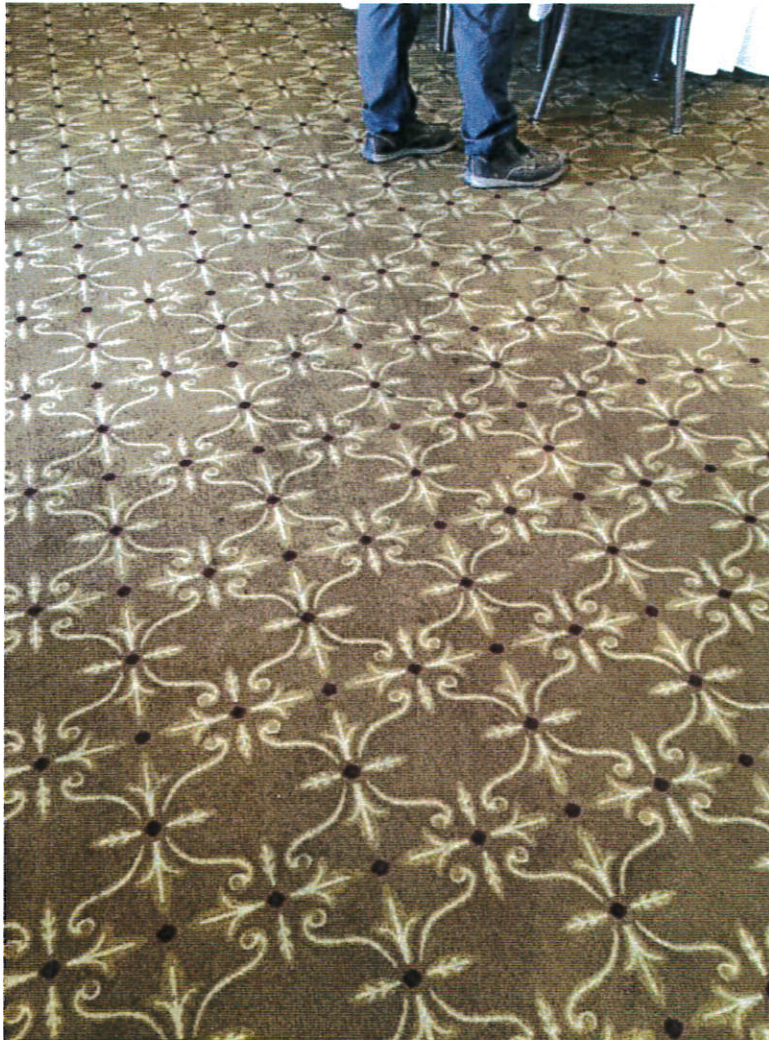
106 106-Pre-Mitigation - Dining Room Date Taken: 12/26/2022 (Zone 1) 3
