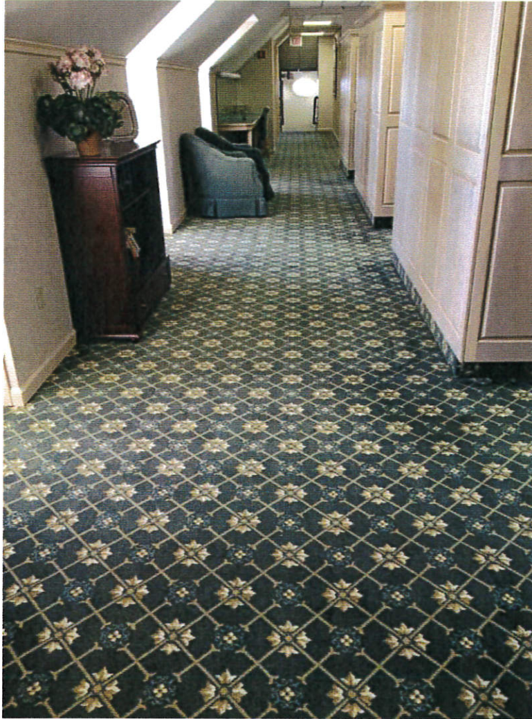
156 156-Pre-Mitigation - Locker room Date Taken: 12/26/2022 (Zone 1)
