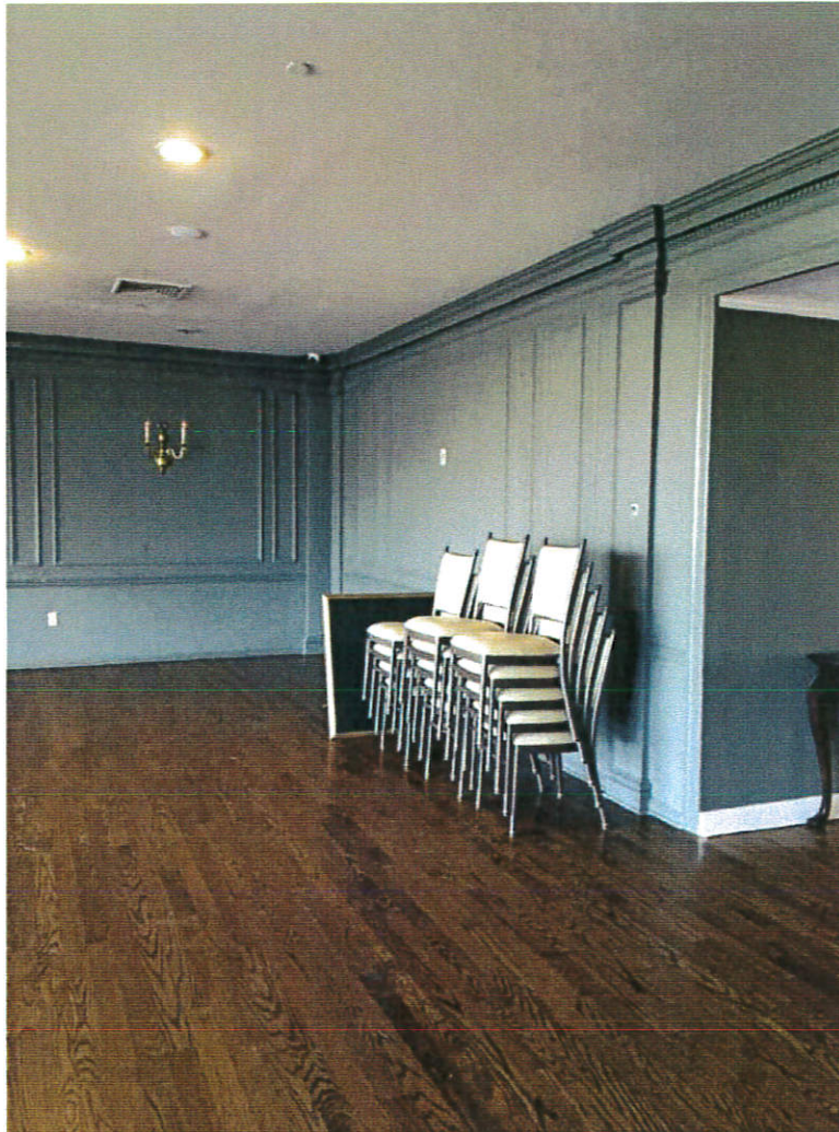
91 91-Pre-Mitigation - Ball room Date Taken: 12/26/2022 (Zone 2) 11
