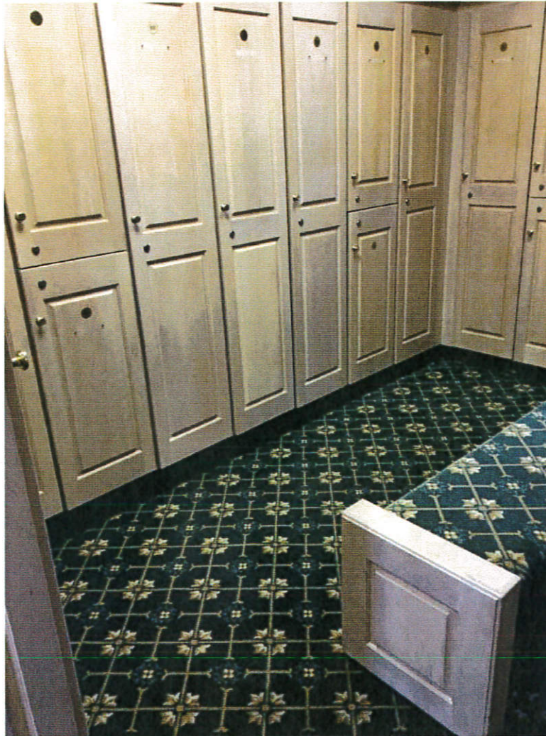
147 147-Pre-Mitigation - Locker room Date Taken: 12/26/2022 (Zone 1) 17
