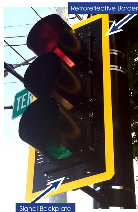
Signal backplate framed with a retroreflective border. Source: FHWA
