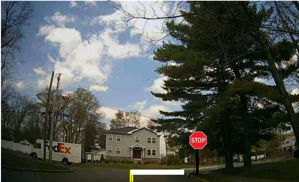
FIGURE 4b – STOP Sign Installation at Ash Avenue & Hillcrest Avenue
