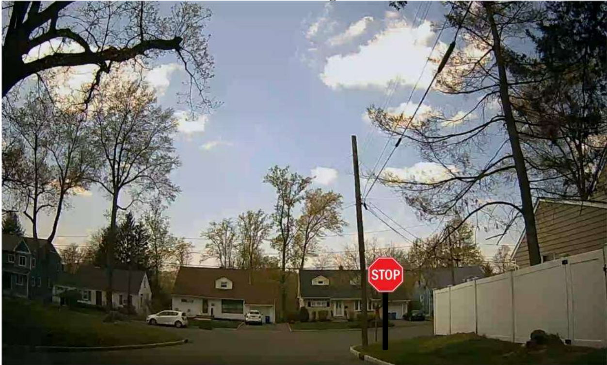
FIGURE 4 – STOP Sign Installation
