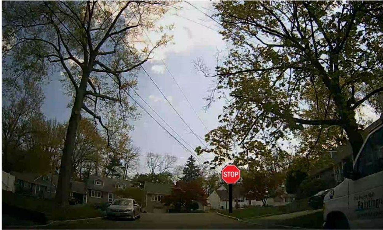
FIGURE 4 – STOP Sign Installation
