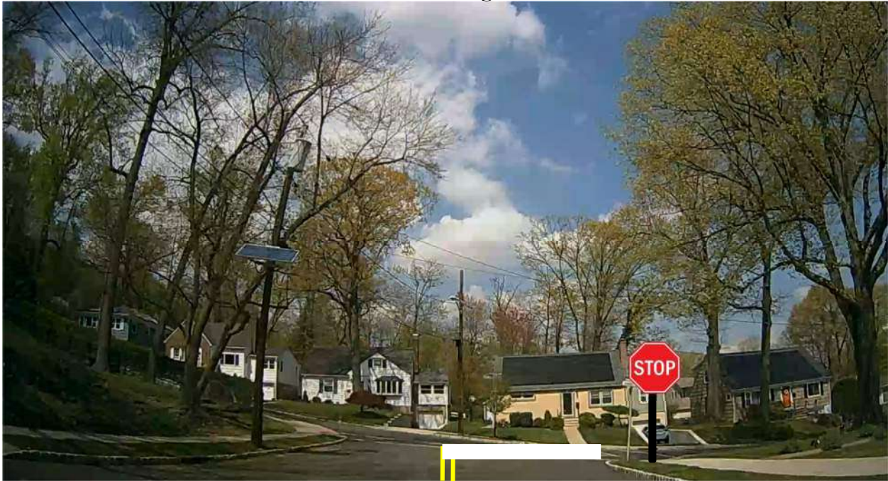
FIGURE 4 – STOP Sign Installation
