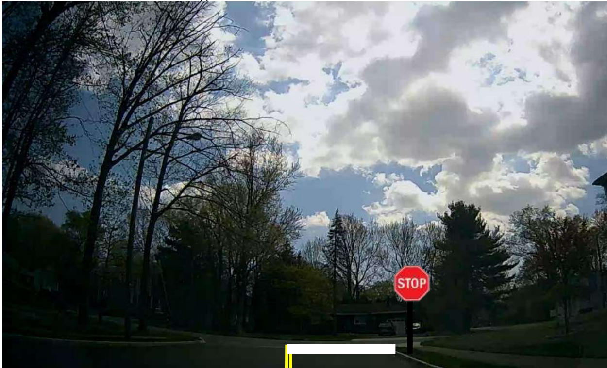
FIGURE 4a – STOP Sign Installation at Knollwood Drive & Hillcrest Avenue
