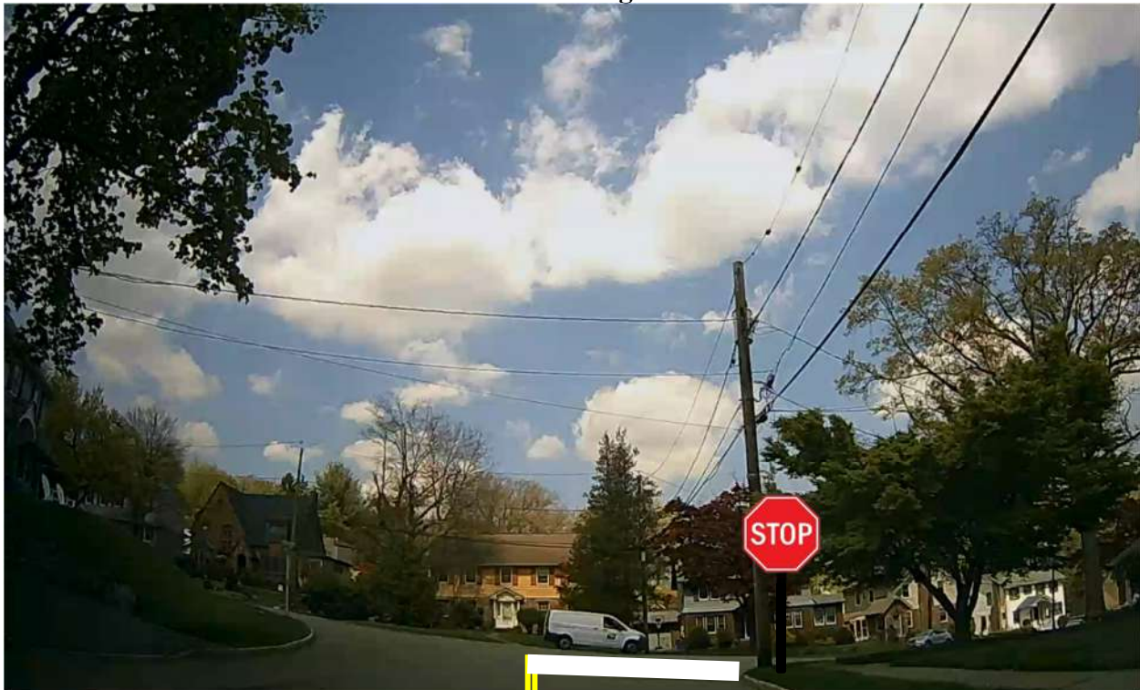
FIGURE 4 – STOP Sign Installation
