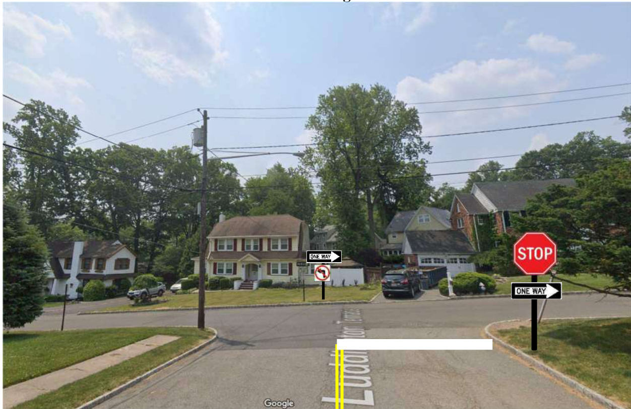
FIGURE 4 – STOP Sign Installation
