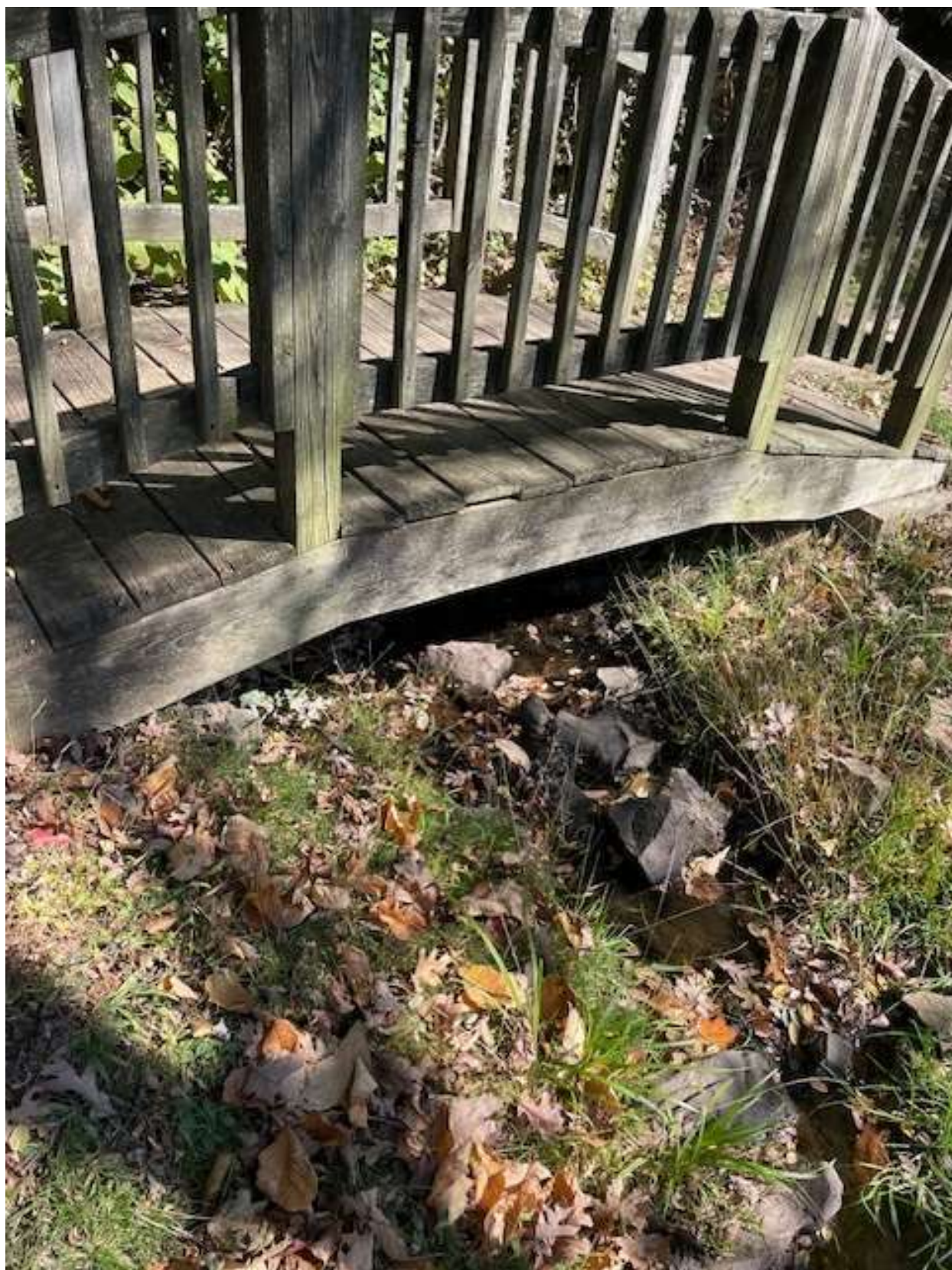
WOODEN PEDESTRIAN BRIDGE
