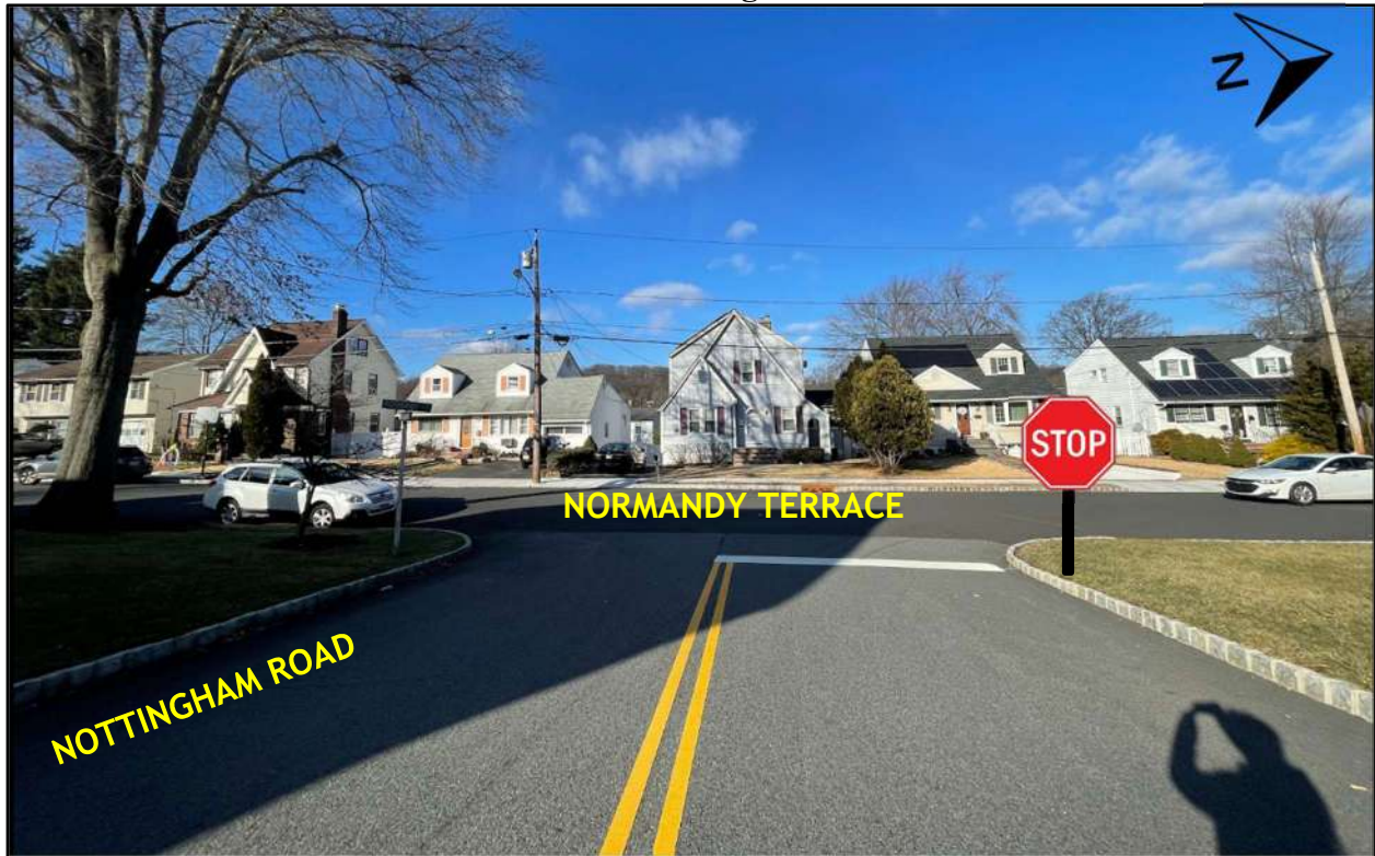
FIGURE 4 – STOP Sign Installation
