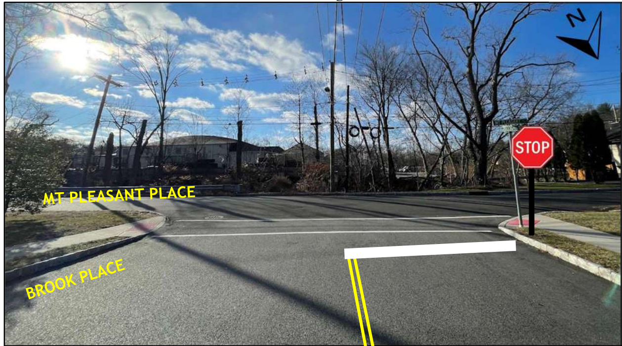
FIGURE 4 – STOP Sign Installation
