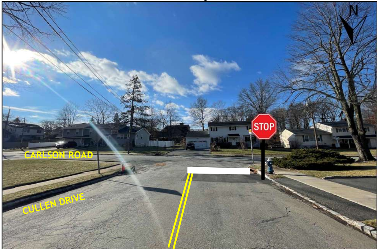
FIGURE 4 – STOP Sign Installation
