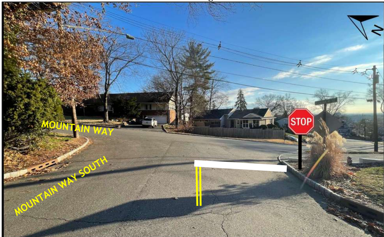
FIGURE 4 – STOP Sign Installation
