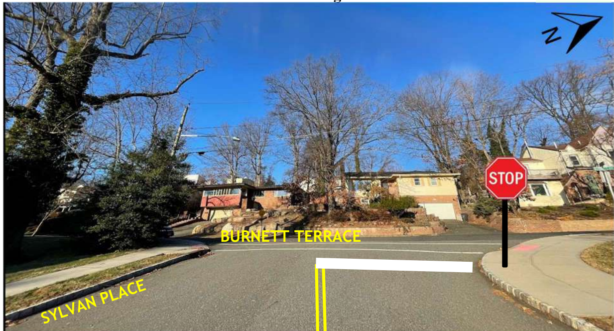
FIGURE 4 – STOP Sign Installation
