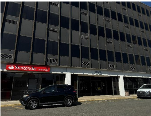
Figure 6: The office building's primary entrance
