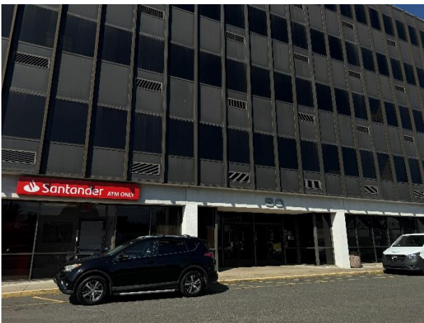
Figure 6: The office building's primary entrance
